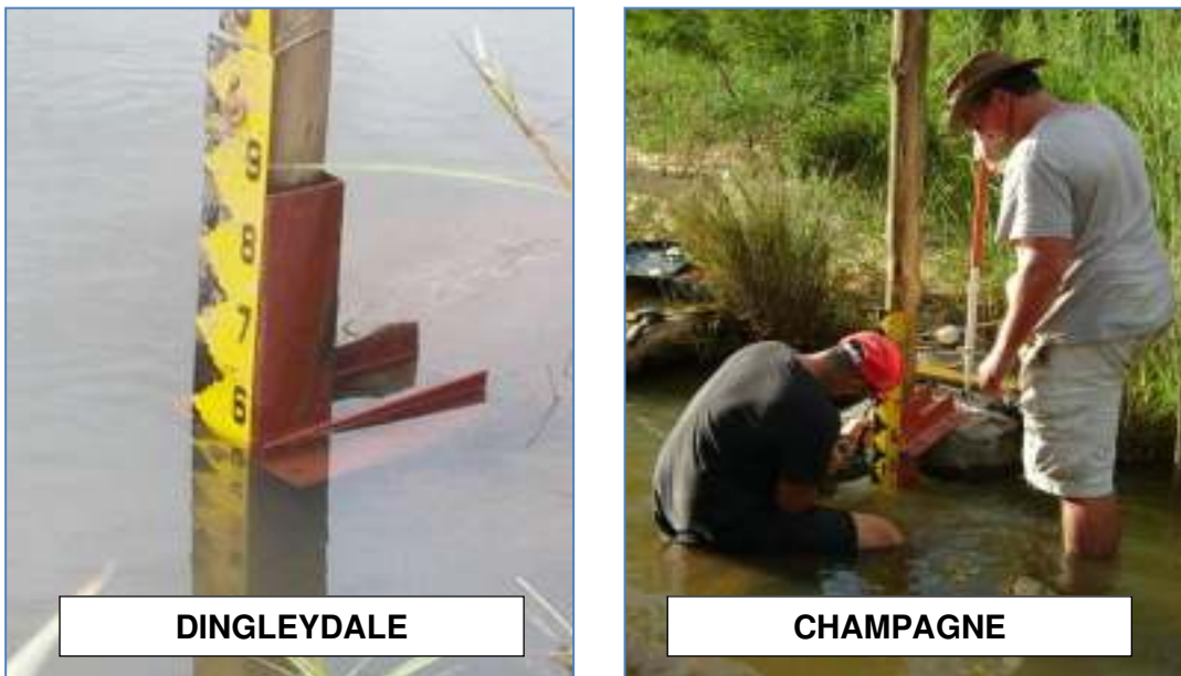
Figure 9.7 Installation of River Flow Gauges
