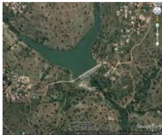
Figure 11: Mahleve Dam and its outflow
