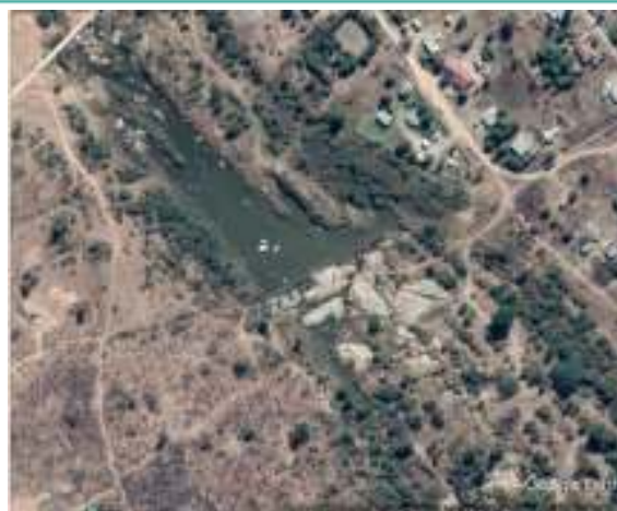
Figure 16: damming of the River, aided by a large weir / construction (Edinburgh Weir)
