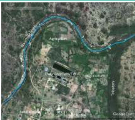
Figure 33: Nwarhele River at Dwarloop WWTW
