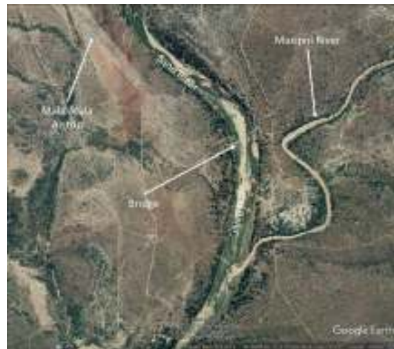
Figure 63: Sand River downstream of Mala-Mala
